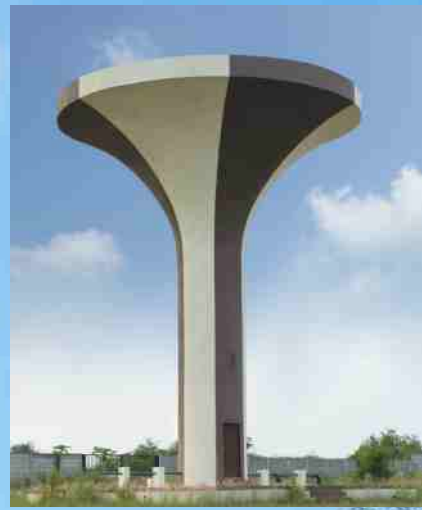
Overhead water supply tank
